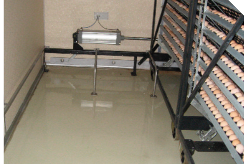
Figure 1 Standing water on the floor of a single stage setter at the end of the sealed period.
