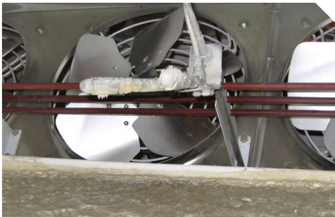
Figure 1 Blocked spray nozzles in setter No. 6
