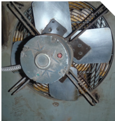
Figure 1 Clean fan blades, well centred fan and correct height.
