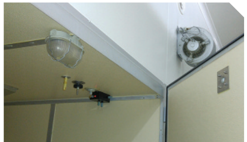
Figure 1 A hole drilled in the door and protected with a metal plate allows the insertion of the calibration probe close to the temperature sensor.
