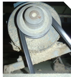
Figure 2 Incorrect fan belt sitting low in the pulley.
