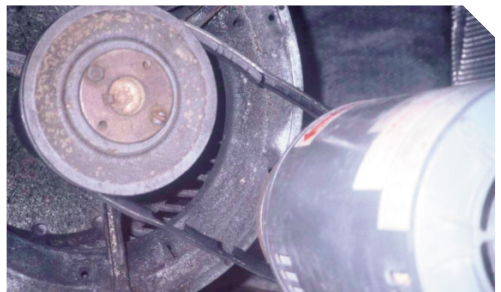
Figure 2 Fan belts should be checked regularly and replaced as necessary – this belt is not fit for use.
