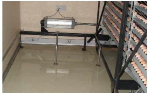
Figure 1 Standing water on the floor of a single stage setter at the end of the sealed period.
